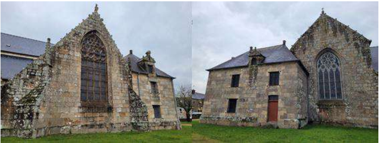
Façade sud (transept)
